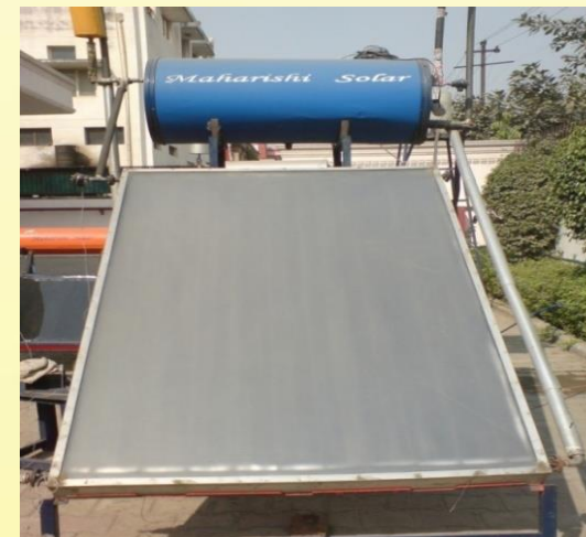
[Solar Water Heating System]
